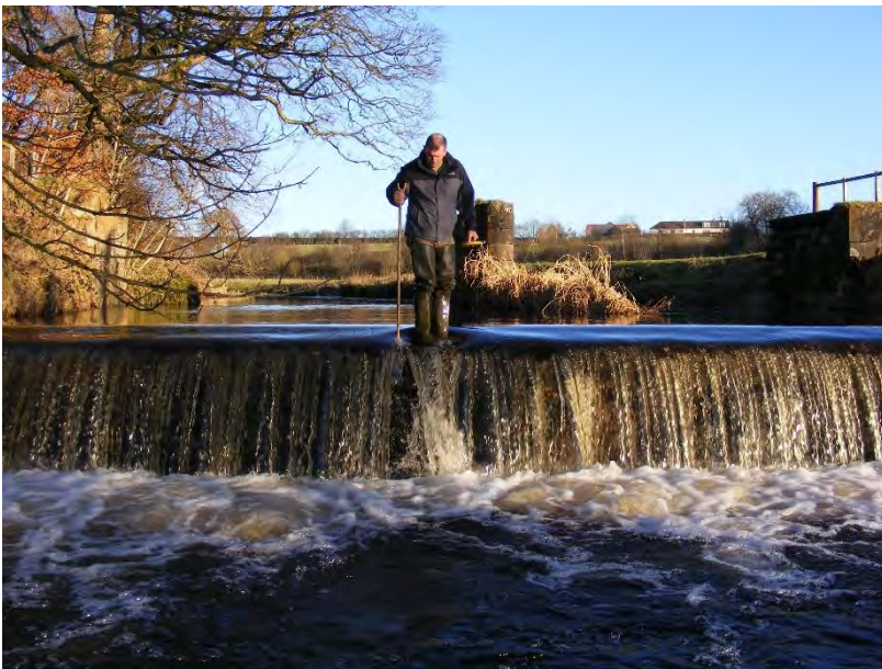
Figure 28: Lainshaw weir - Annick Water
